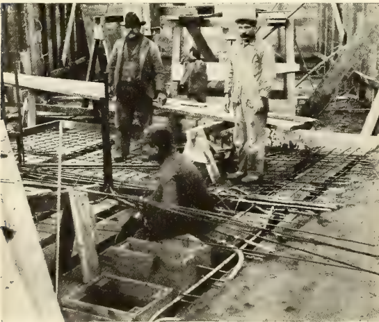
FIG. 3. SHOWING HOW THE FLOORS ARE REINFORCED BY IRON RODS BEFORE THE CONCRETE IS POURED OVER THEM.
